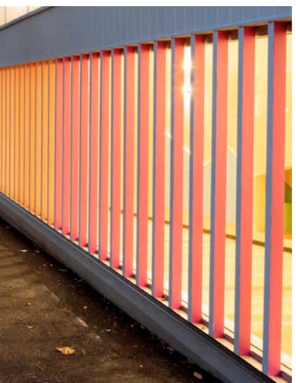
SCR1 Vertical coloured batten screening. Colours interspersed
