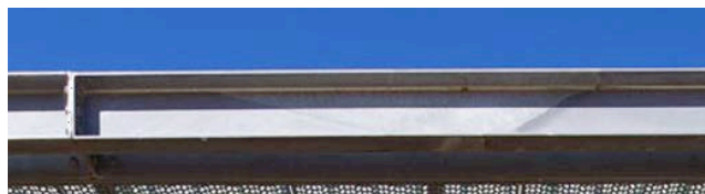
MR Metal roof steel frame
